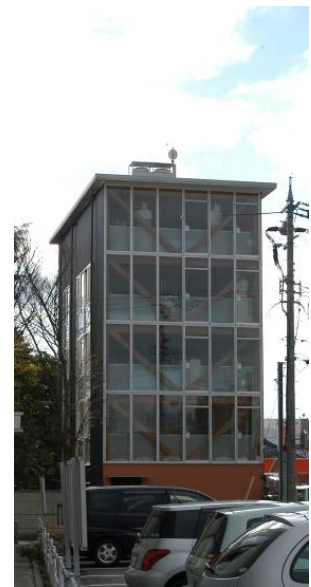
Photo.1 External view of Kanazawa M Bldg.
